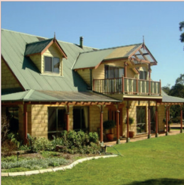
Timbercrete is a lightweight composite masonry material available in bricks, blocks, panels and pavers.
