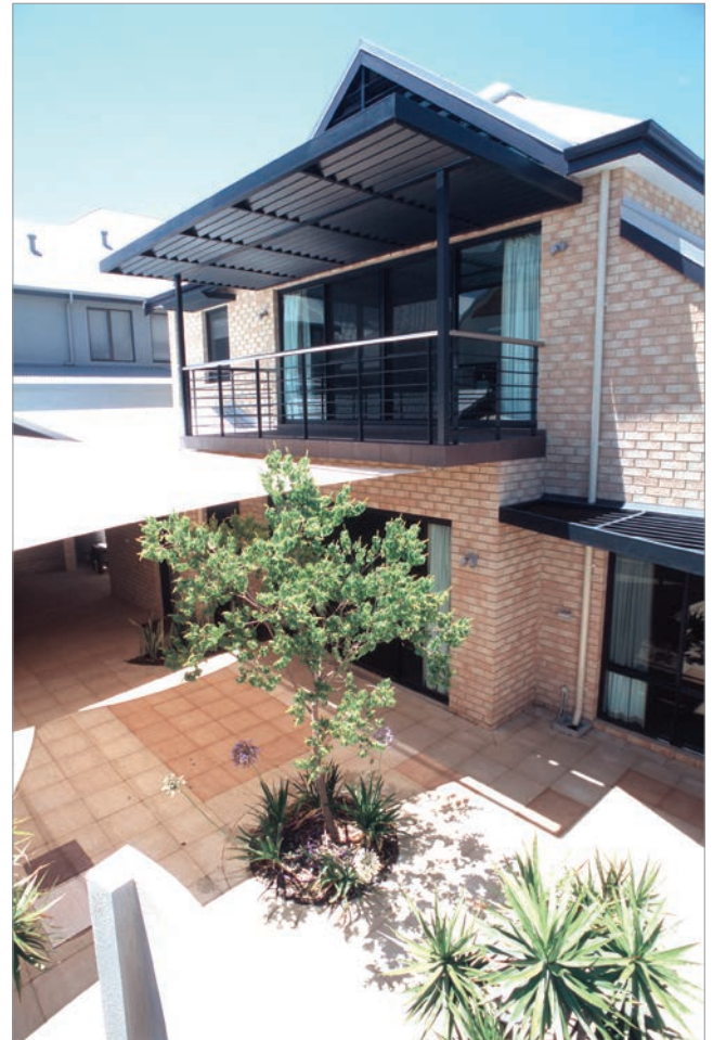
The walls of this house are a combination of double brick and reverse brick veneer.
